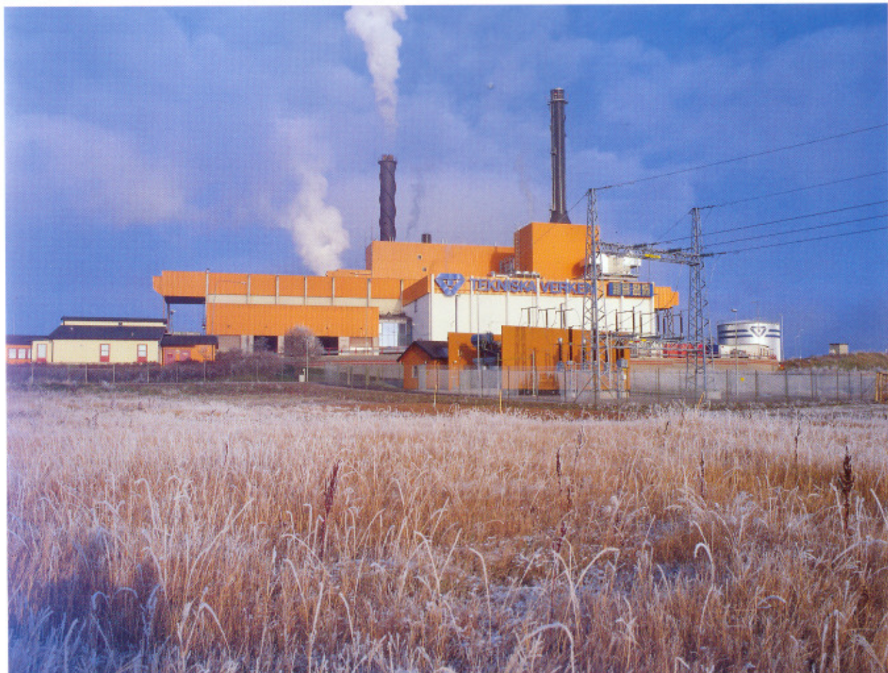
The Gästadsverket works is one of the power plants monitored by the new Cactus system. Gästadsverket is a combined power and heating plant, which means it can produce both electric and district heating. The fuel it uses is household waste – 200,000 tonnes from more than 500,000 people. The amount of energy produced is equivalent to about 50,000 tons of oil per year.
